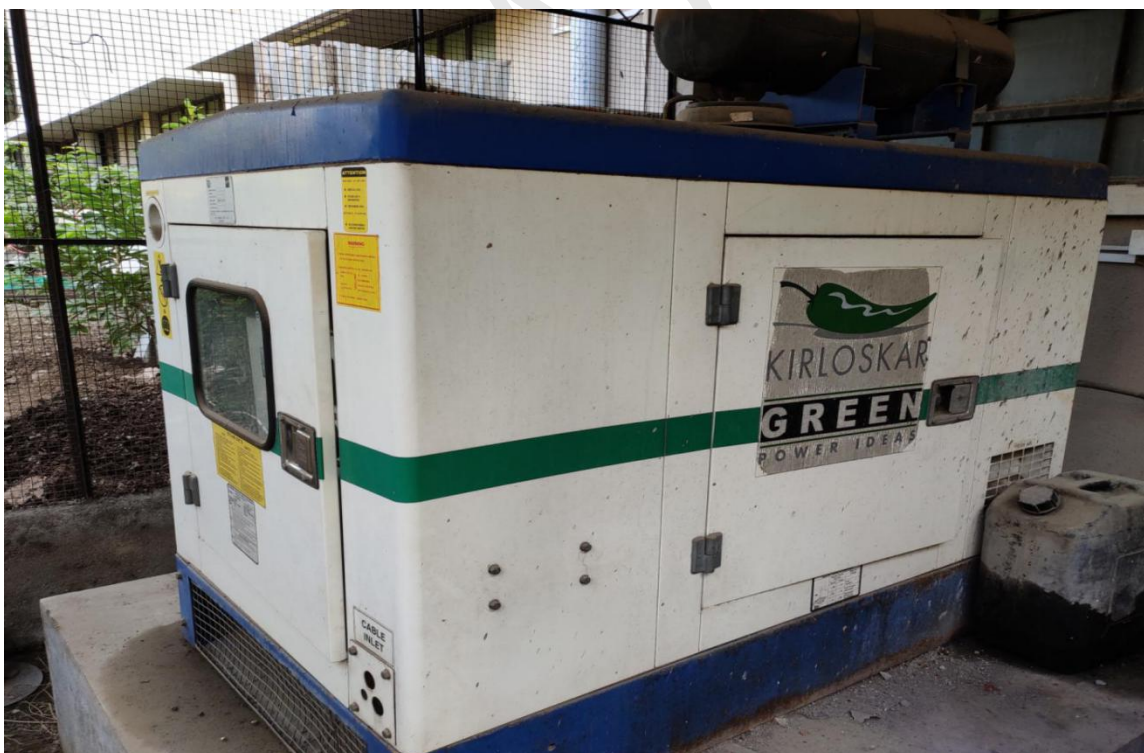
Diesel Generator (15kVA)
