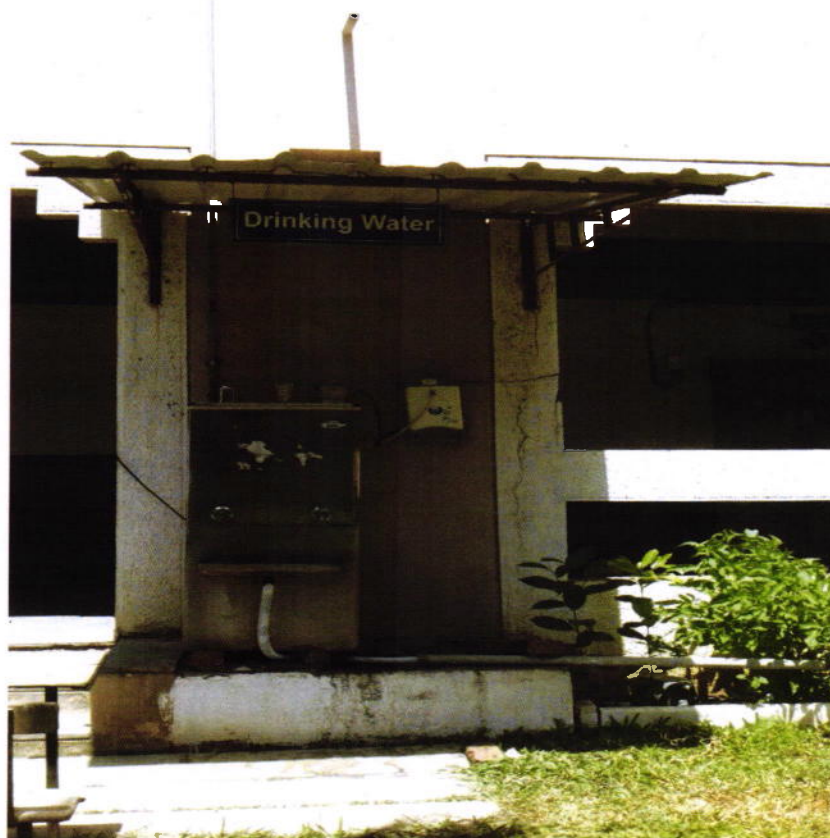
Water Sampling for Testing Purpose
