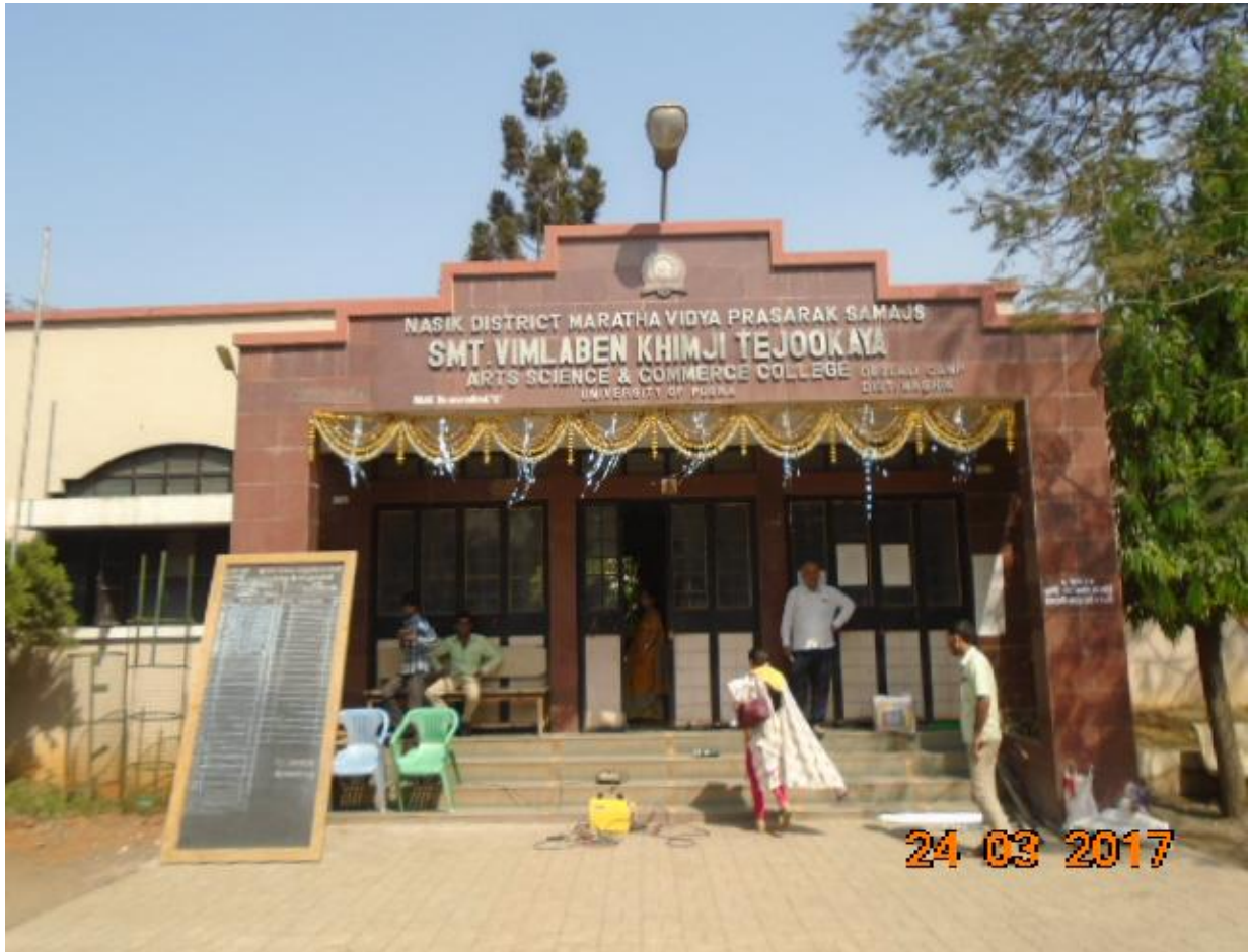
College Entry Gate
