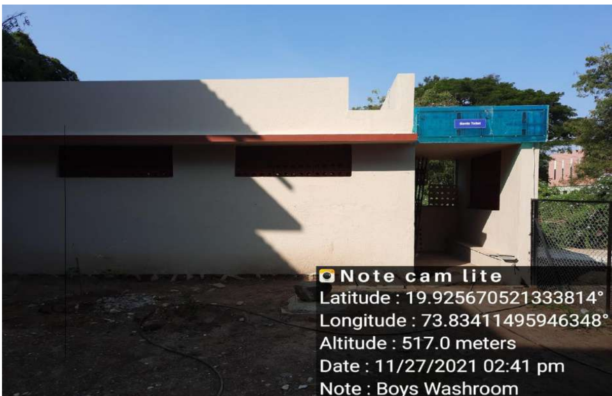
Figure 16. Boys Wash Rooms
