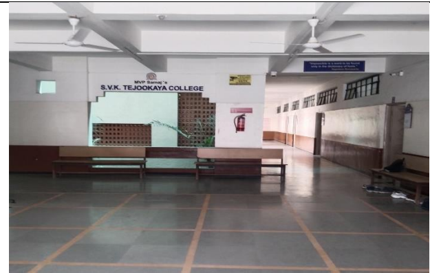
Ground floor passge Front side
